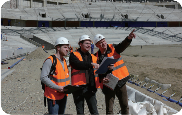
Huawei delivered its Indoor Connected Solution (ICS) to a football stadium in Russia.
